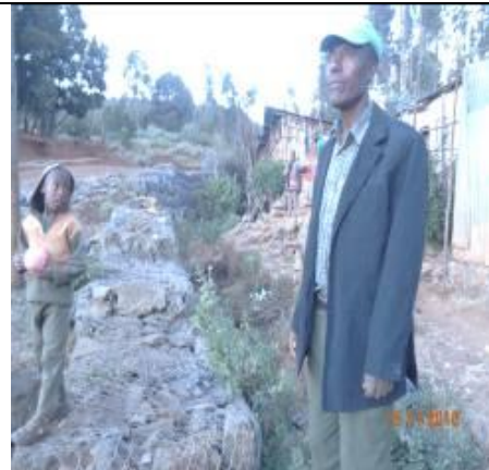
Household protected by gabion walls, Yekai 01 Woreda Addi Ababa City
