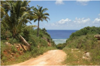
Minor adjustments to Mangaia Harbour dramatically improved its resilience to natural disasters. Photo: Andrea Egan
